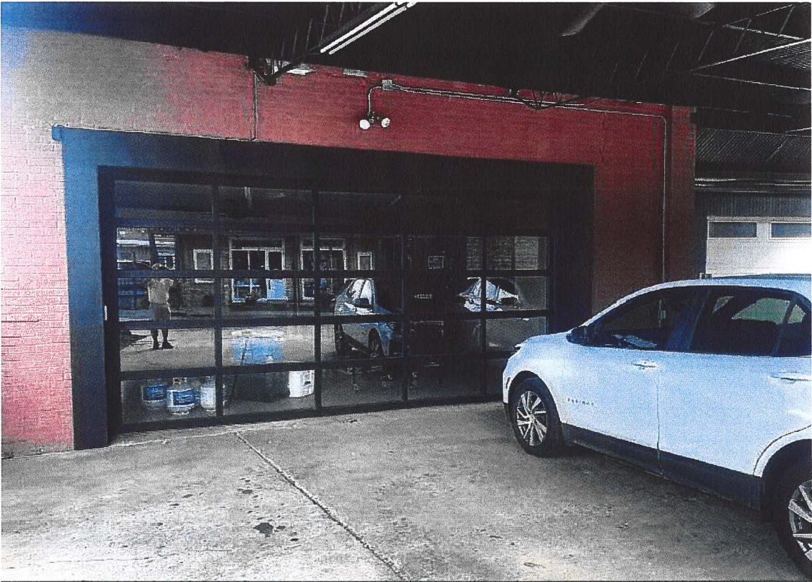
Overhead door we will be matching other doors to
