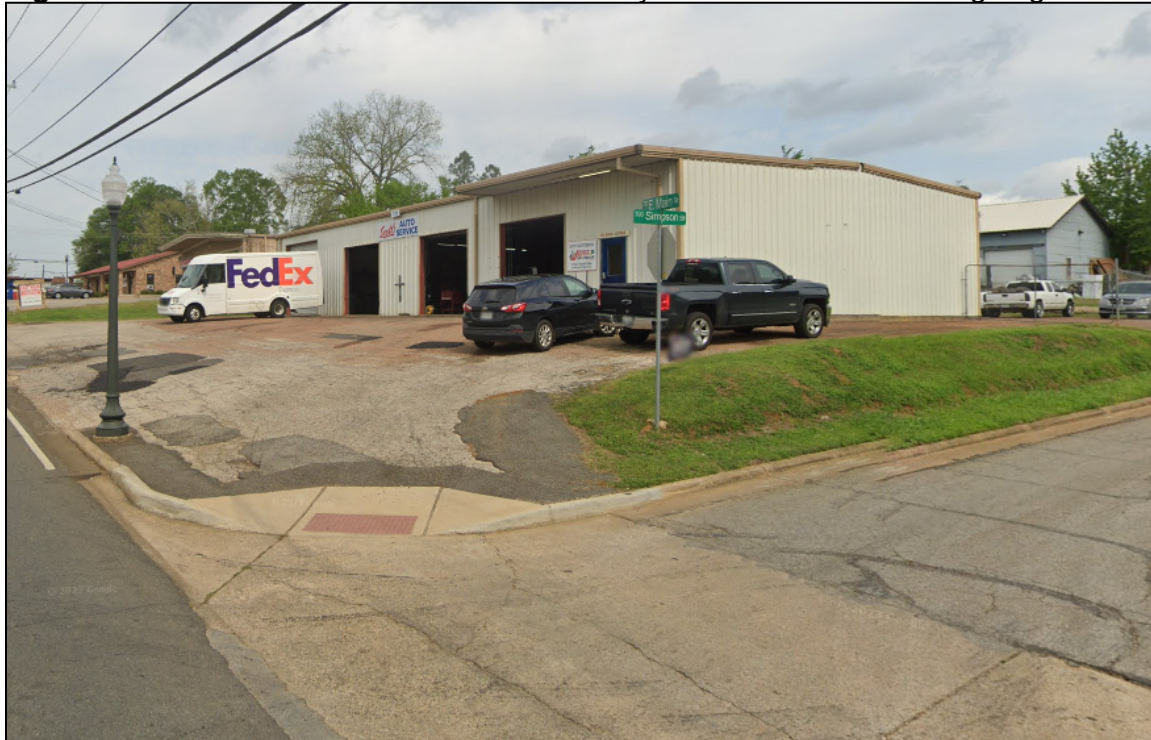
Figure 7 ---725 E Main Street---late 1970s to early 1980s-built commercial garage
