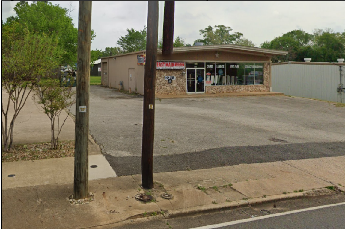
Figure 8 ---711 E Main Street---ca. late-1970s to early-1980s-built commercial warehouse
