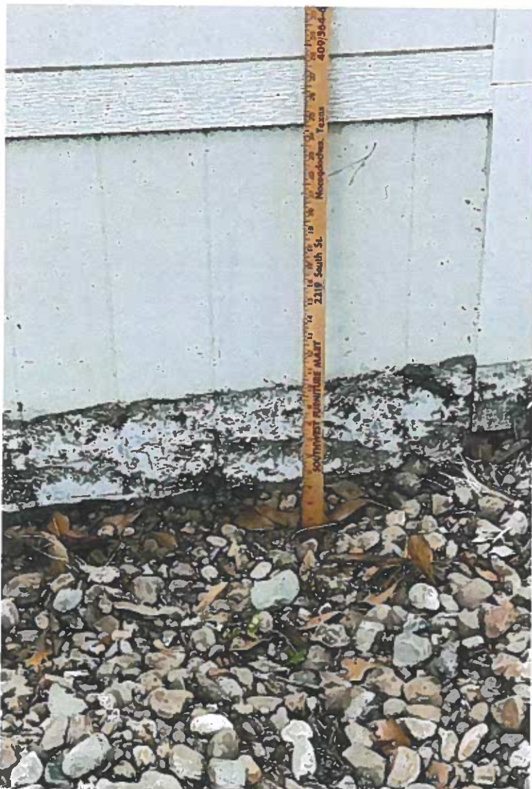
PICTURES SHOW HOW MUCH SEDIMENT WAS DEPOSITED AGAINST THE SIDE OF THE GARAGE.
