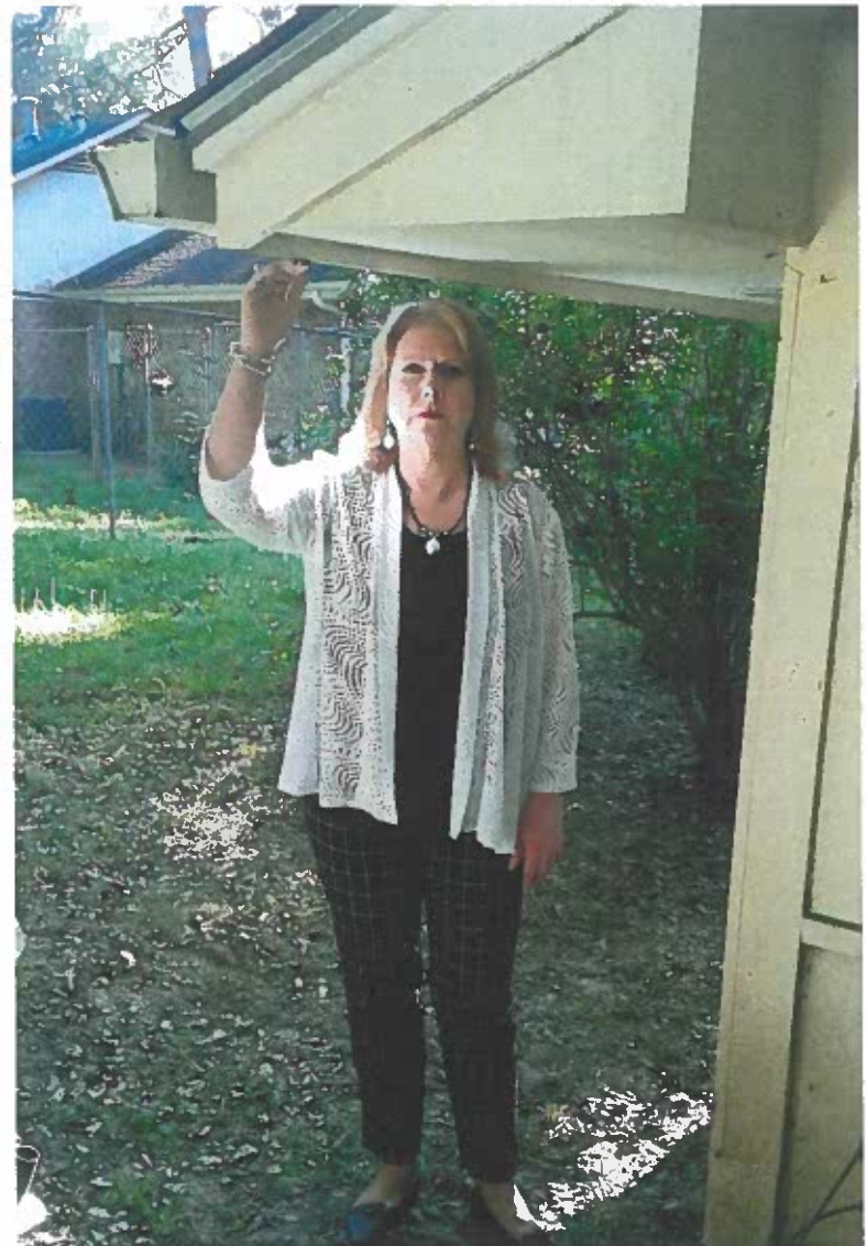
BACK OF GARAGE SHOWING AMT. OF DEPOSITED SAND
