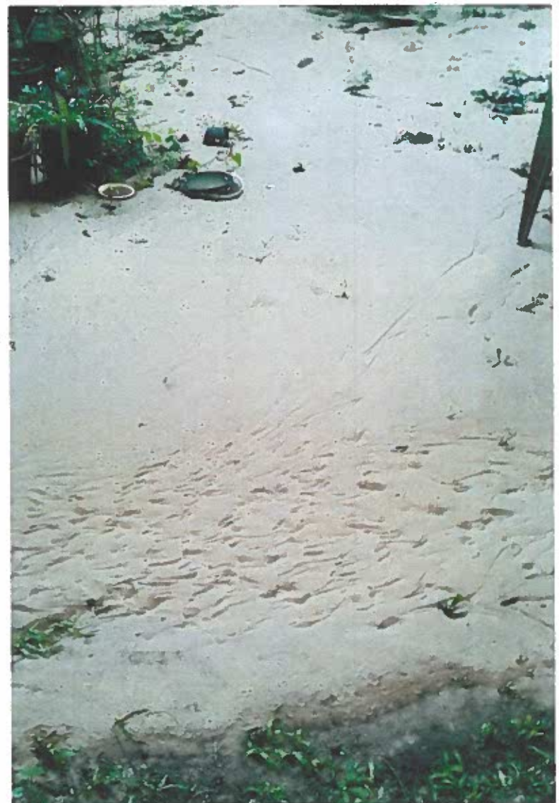
BRICK PATIO COMPLETELY COVERED IN SAND WASHED DOWN FROM FIELD OF APPLEBY SAND RD./EAST AUSTIN
