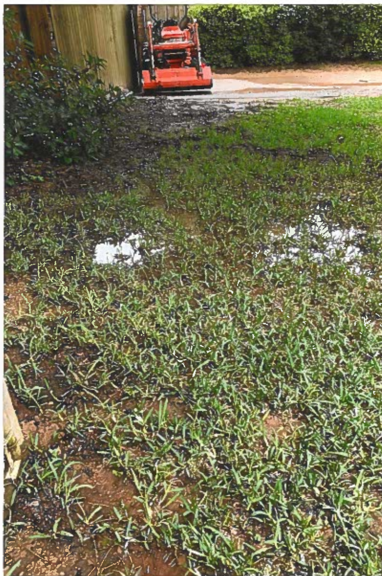
NOTE AMOUNT OF SAND ON driveway WE NEVER HAD A PROBLEM WITH STANDING WATER
