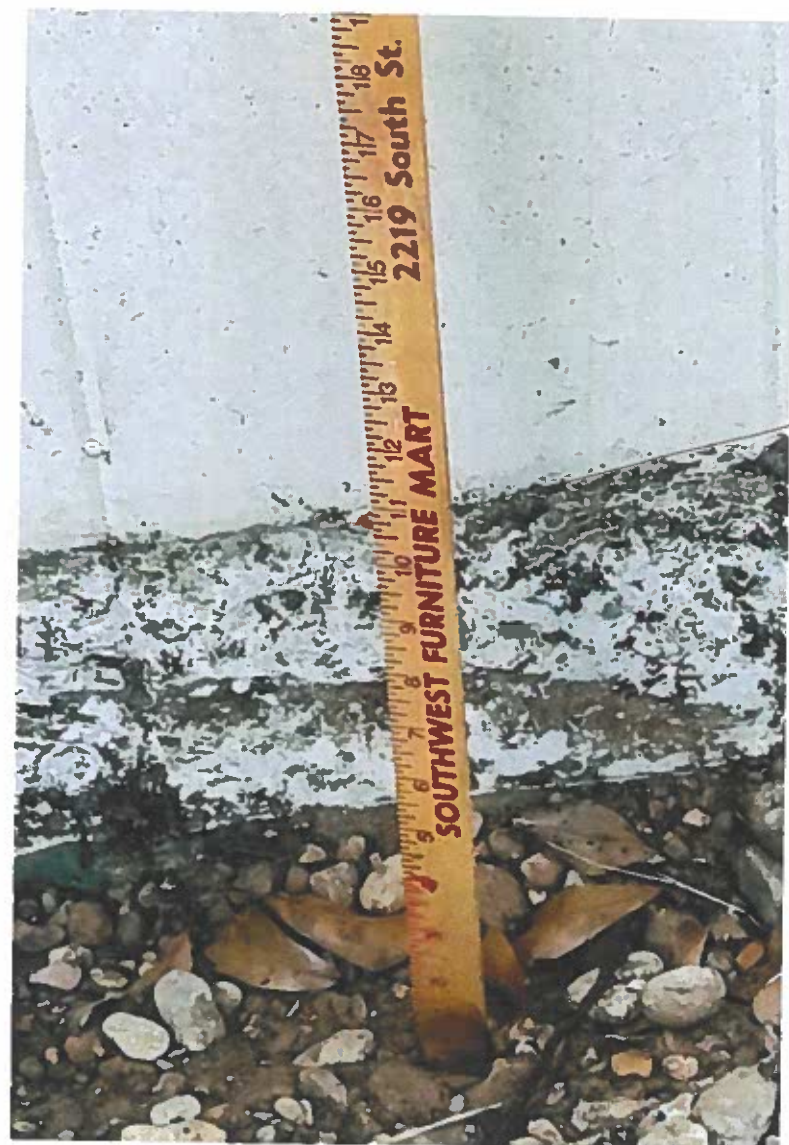
PICTURES SHOW HOW MUCH SEDIMENT WAS DEPOSITED AGAINST THE SIDE OF THE GARAGE.
