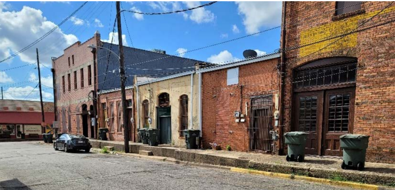
Above ground alley utility in Downtown Commerce Alley
