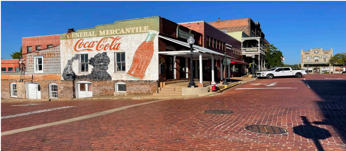
Southeast corner of Downtown square showing 1915 utility manholes.
