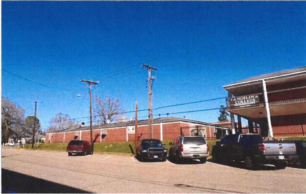
302 Hughes (Cafeteria) Rear Photograph by Ryan Gullett, August 2010
