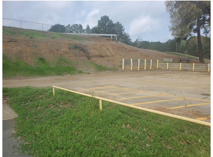
South view - Shore protection
