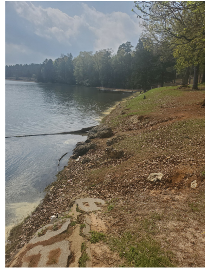
South view - Shore protection
