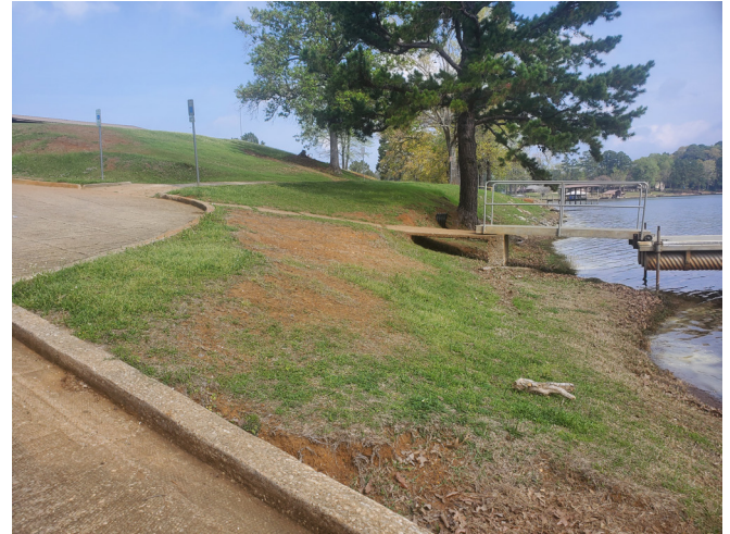
NNW view - Existing pier access
