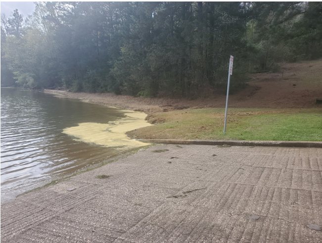
South view - Existing ramp
