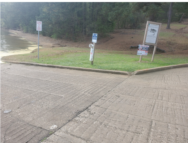
SE View - Existing ramp
