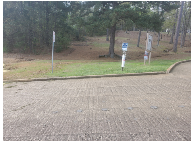
South view - Existing ramp
