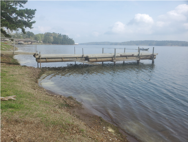
North View - Existing pier to be replaced
