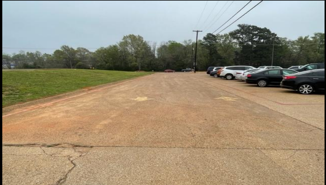
View of shared driveway from apartments
