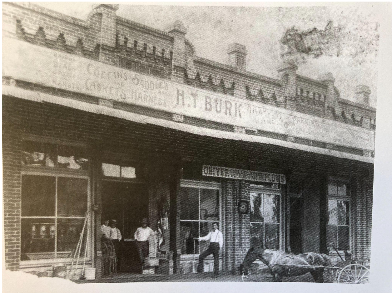
J.W. Powers Building - built ca. 1899, Photo of H.T. Burk Hardware, c. 1910
