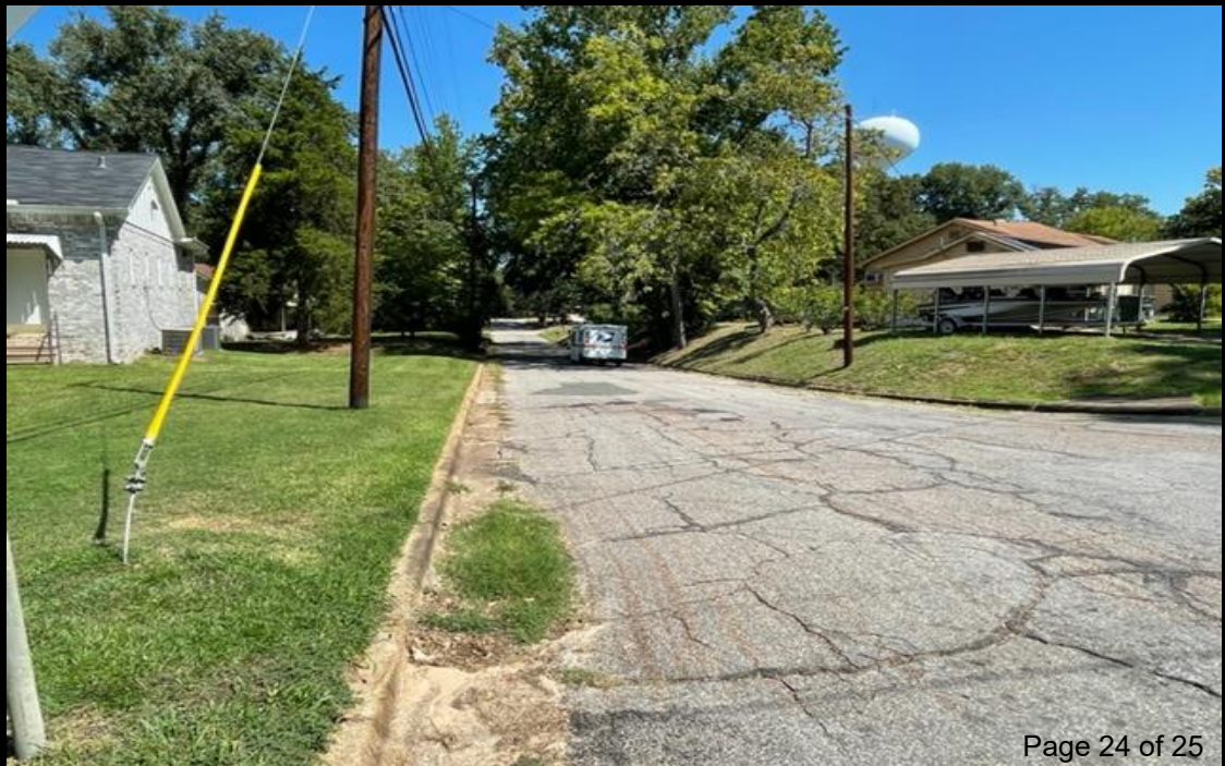
Looking northeast on Lelia St.
