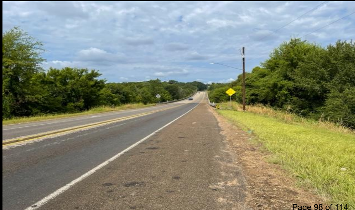
Looking west along W. Austin St.
