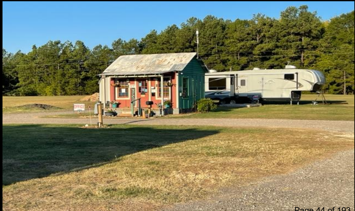
Current office (to be replaced)
