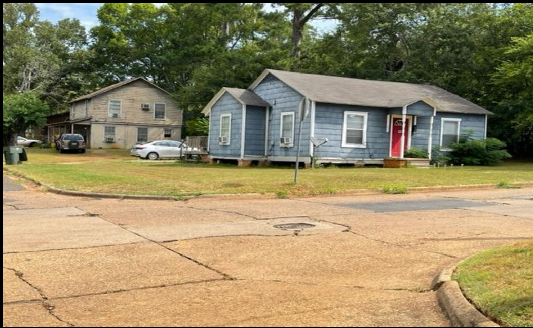
Single family and Duplex houses east of Pearl St.
