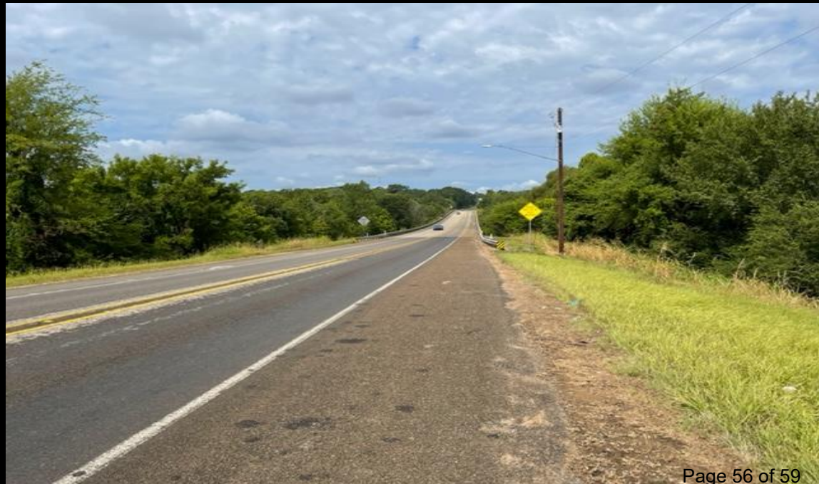
Looking west along W. Austin St.
