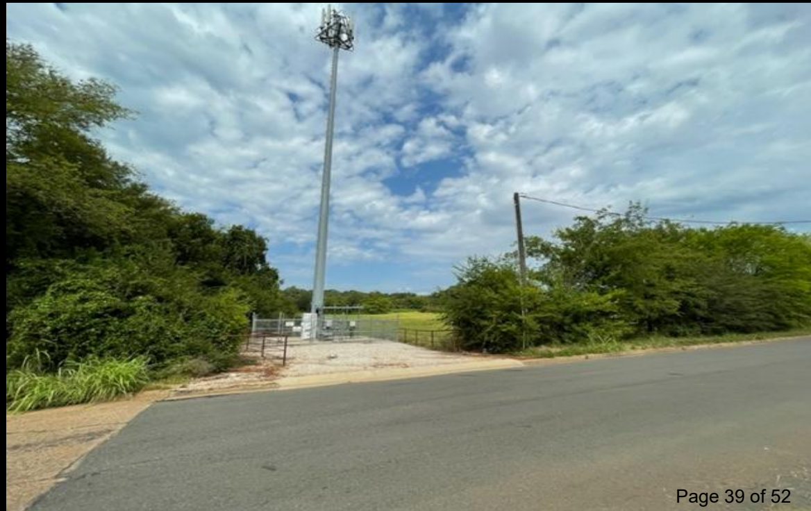
Cell phone tower on the southeast corner of the subject property
