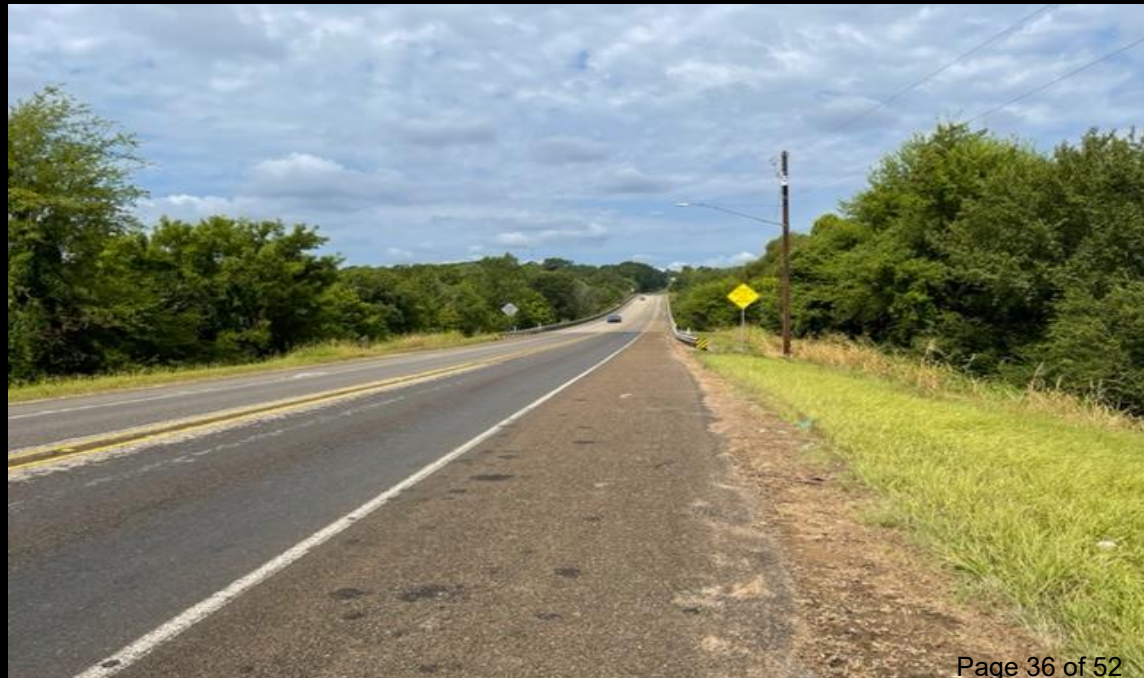
Looking west along W. Austin St.
