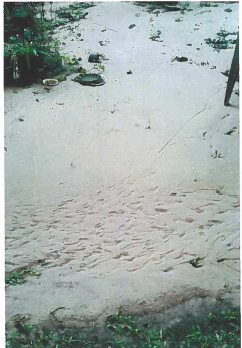
BRICK PATIO COMPLETELY COVERED IN SAND WASHED DOWN FROM FIELD OF APPLEBY SD. RD./E. AUSTIN
