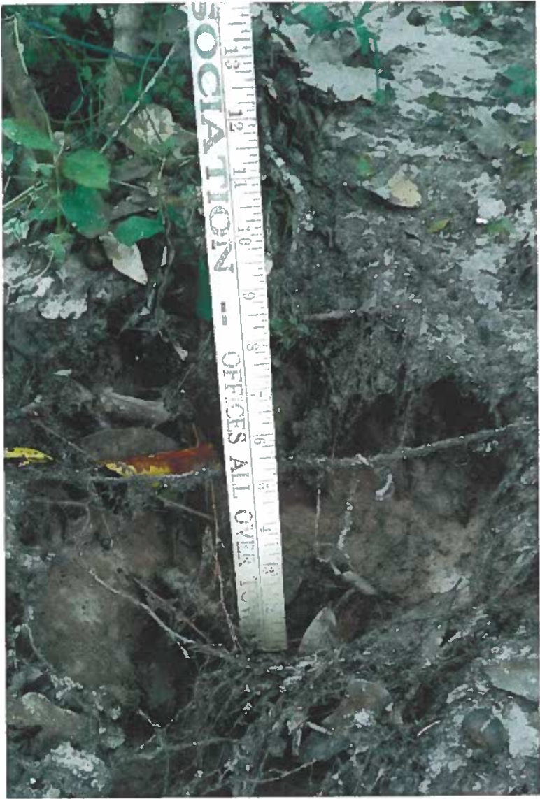
13" WASHOUT - ONE OF MANY
