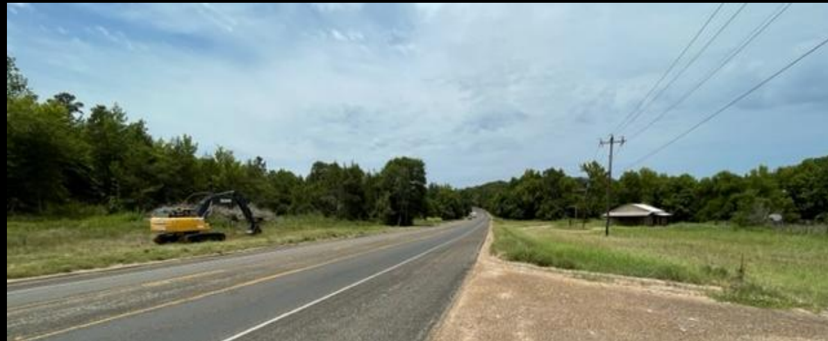
Street view looking north along Old Tyler Rd.
