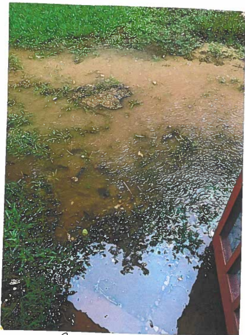
BACK PORCH FLOODING 4-13-2022
