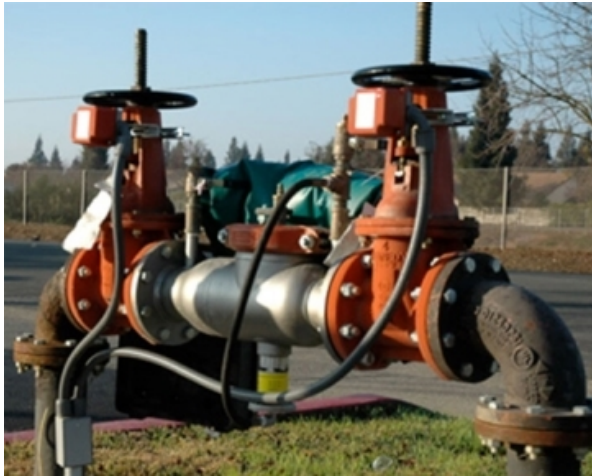
REDUCED PRESSURE ZONE BACKFLOW PREVENTERS
