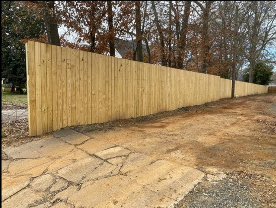
Replacement fence along south property line
