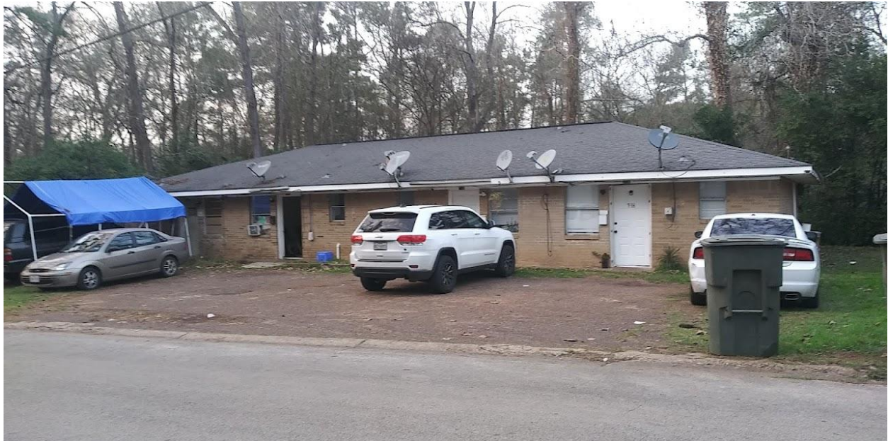
Four plex at 716, 718, 720, 722, Harris Street
