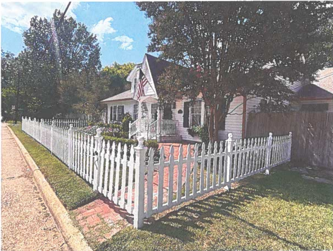
Corner post placed as close to walkway as possible
