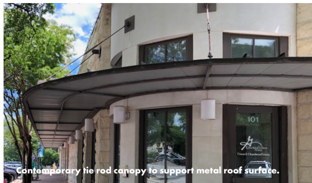
Contemporary tie rod canopy with wood soffit.
