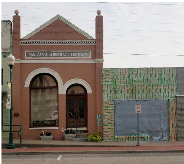
Above: Van Zandt Abstract Company in Canton, Texas carefully removed layers of paint from their front facade using Dumond Peel Away Poultice system.
