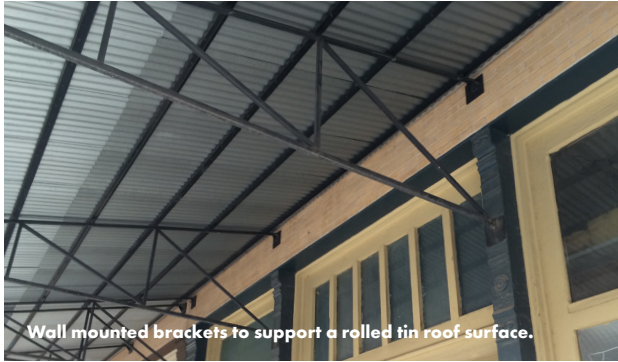
Rolled tin roof surface
