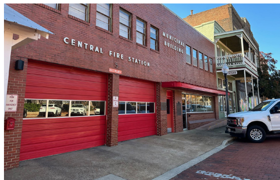
Fire Station No. 5. Source: nactx.us
