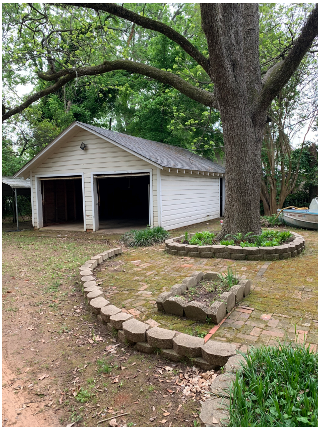
Existing two car garage, to be converted into outdoor living space; walls to be removed to create similar openings on east and west facades
