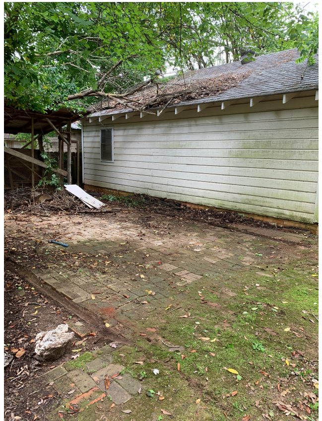
Existing two car garage, to be converted into outdoor living space; walls to be removed to create similar openings on east and west facades
