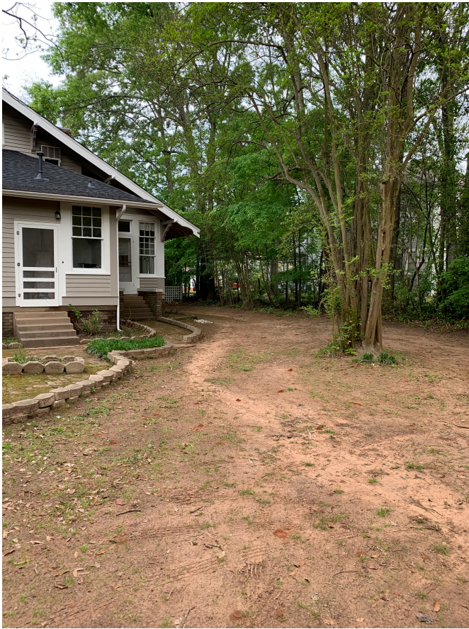
Location of concrete driveway and wrought-iron fence
