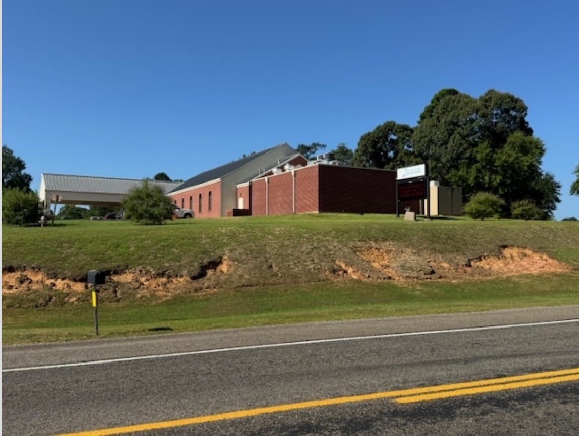
Adjacent Senior Center to the east
