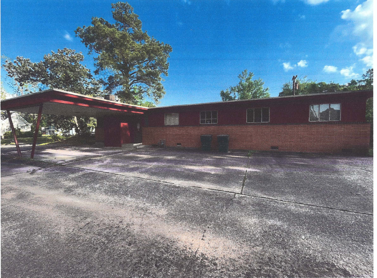
North side of building facing the CE (Christ Episcopal) School
