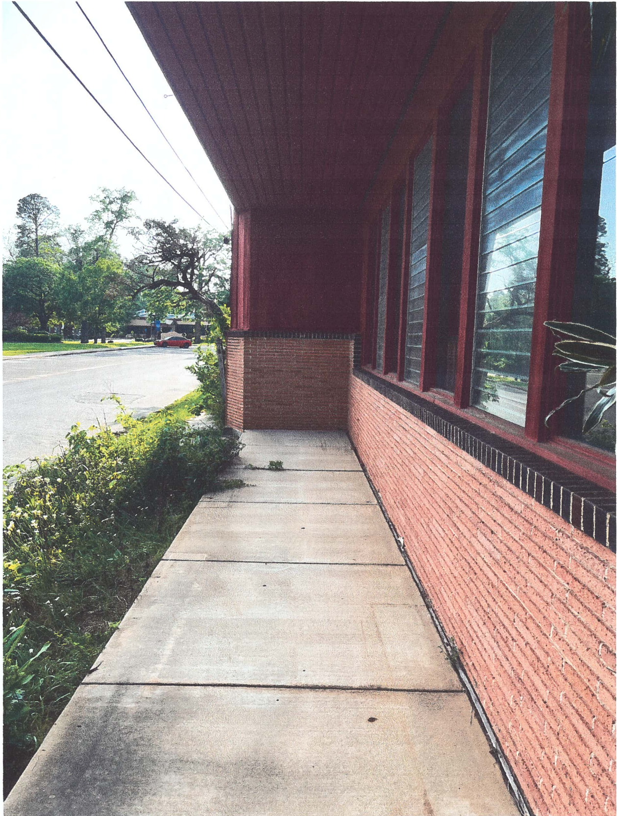
South facing side of building from Bailey St
