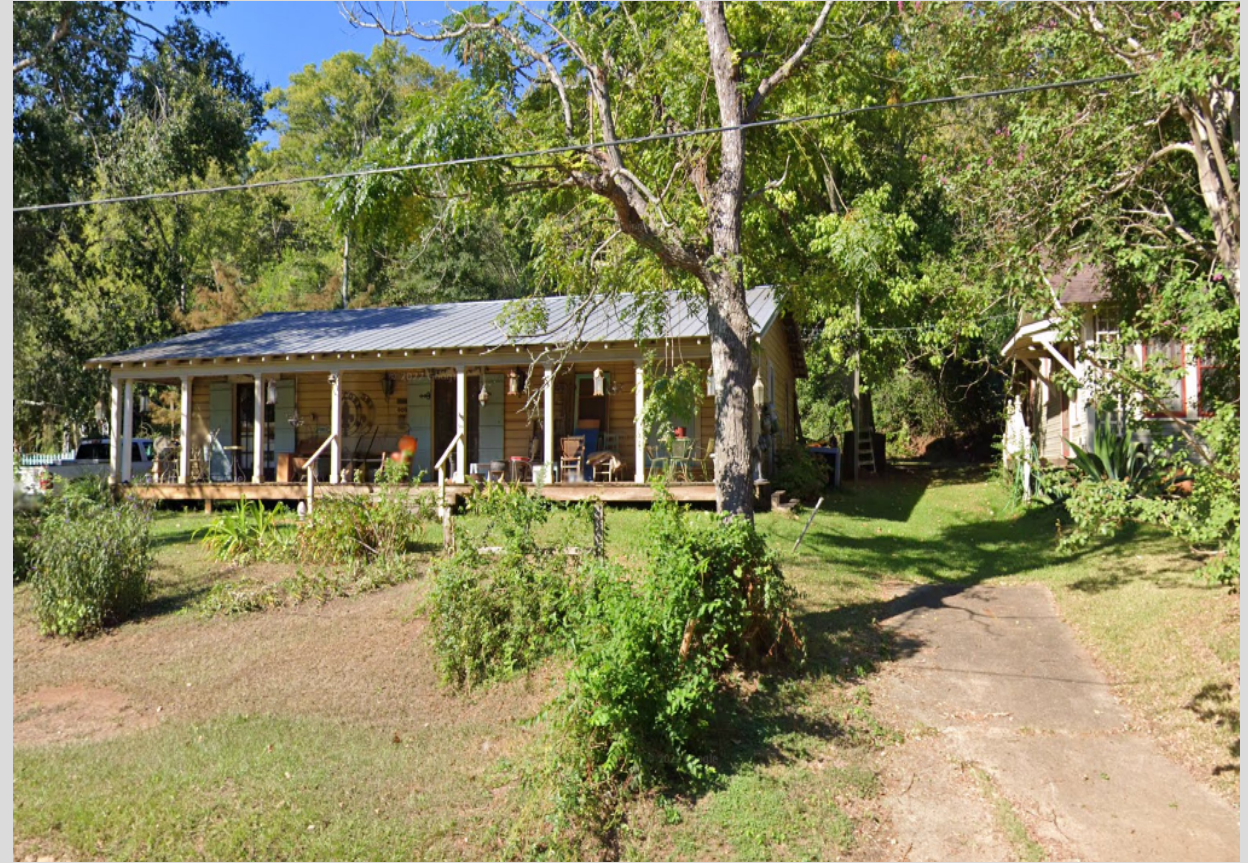
Adjacent residential property to the south
