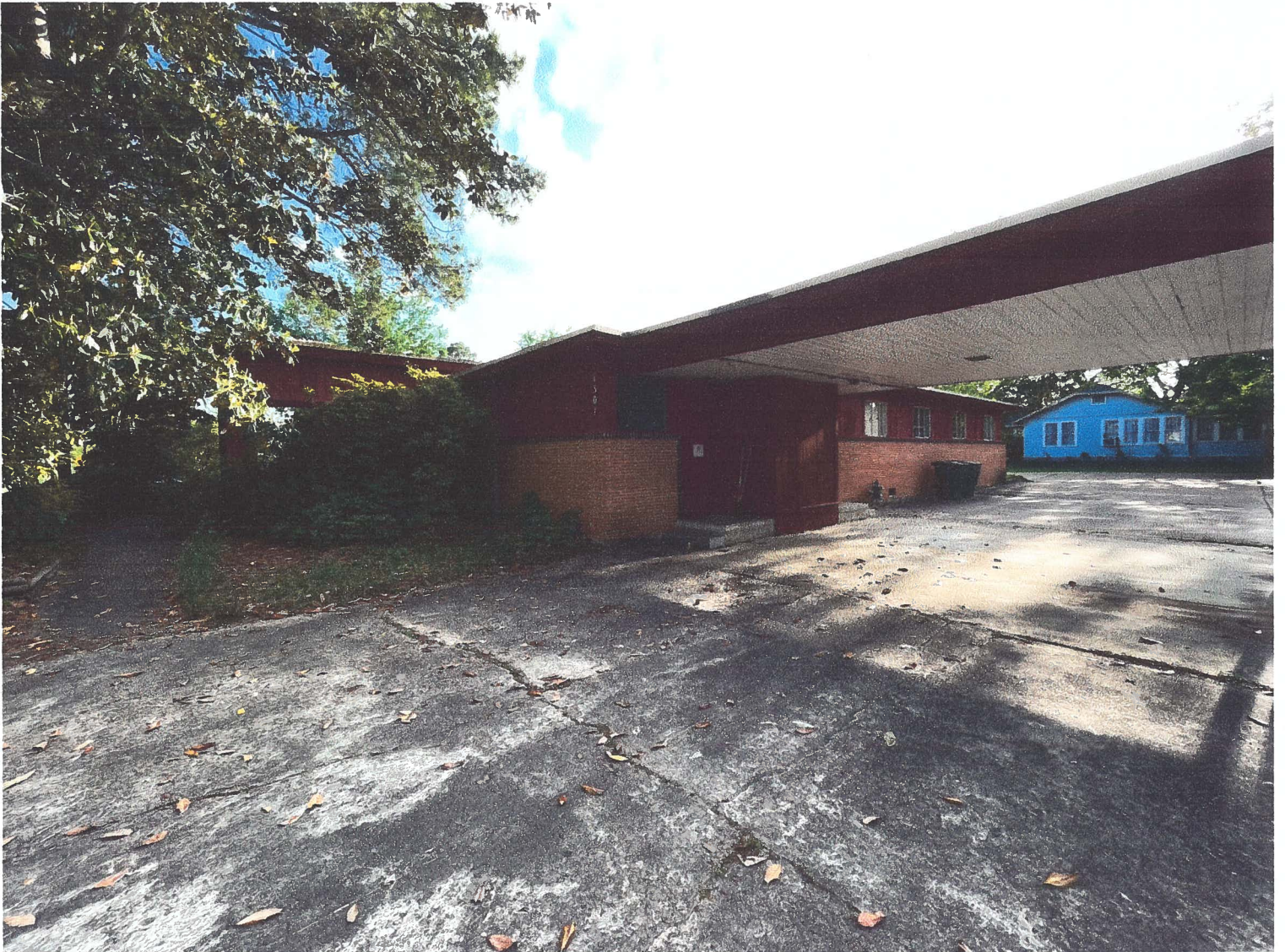
Northern side of building / carport
