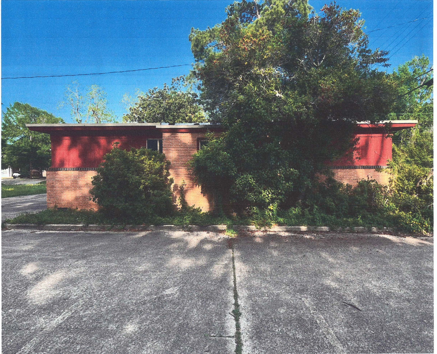
Back of building
