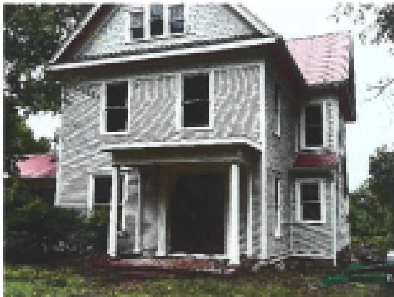
Current view of front as rebuilt to the design when recently purchased.
