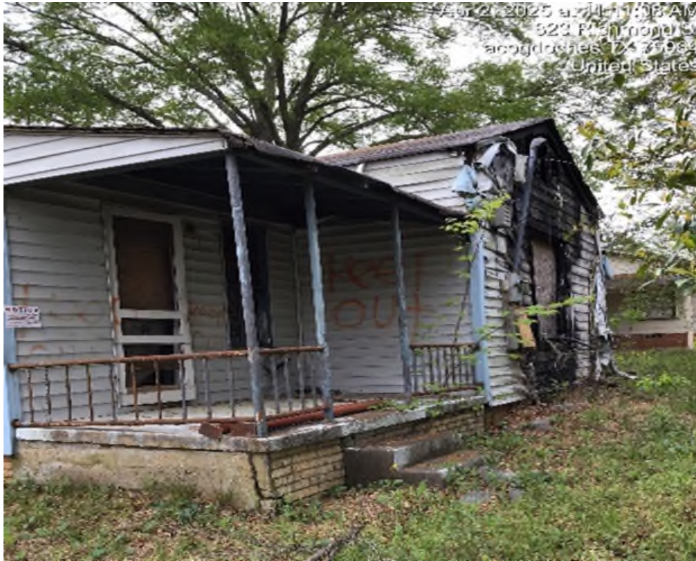
View of structure showing posted notice. Photo taken April 2, 2025.
