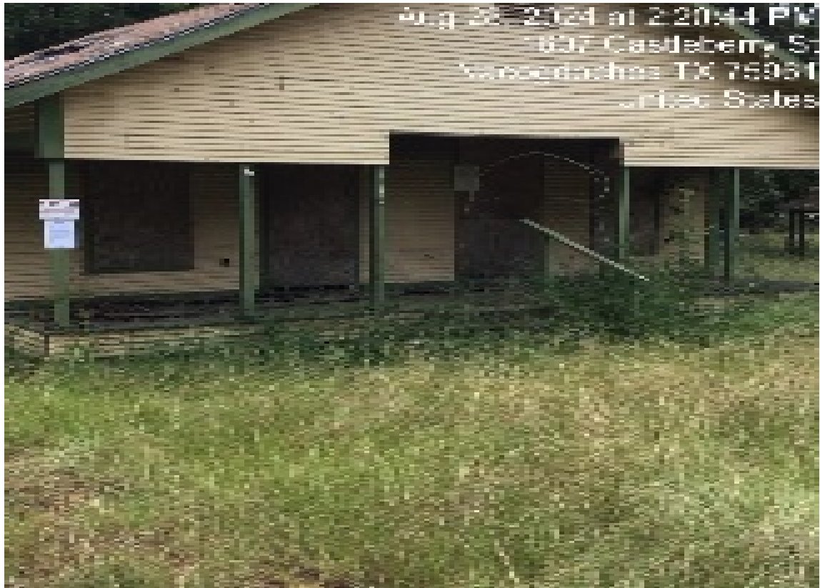
View of structure showing posted notice. Photo taken August 2024.
