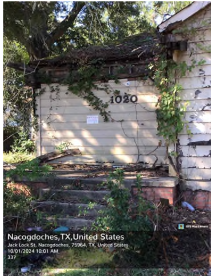
View of structure showing posted notice. Photo taken October 1, 2024.
