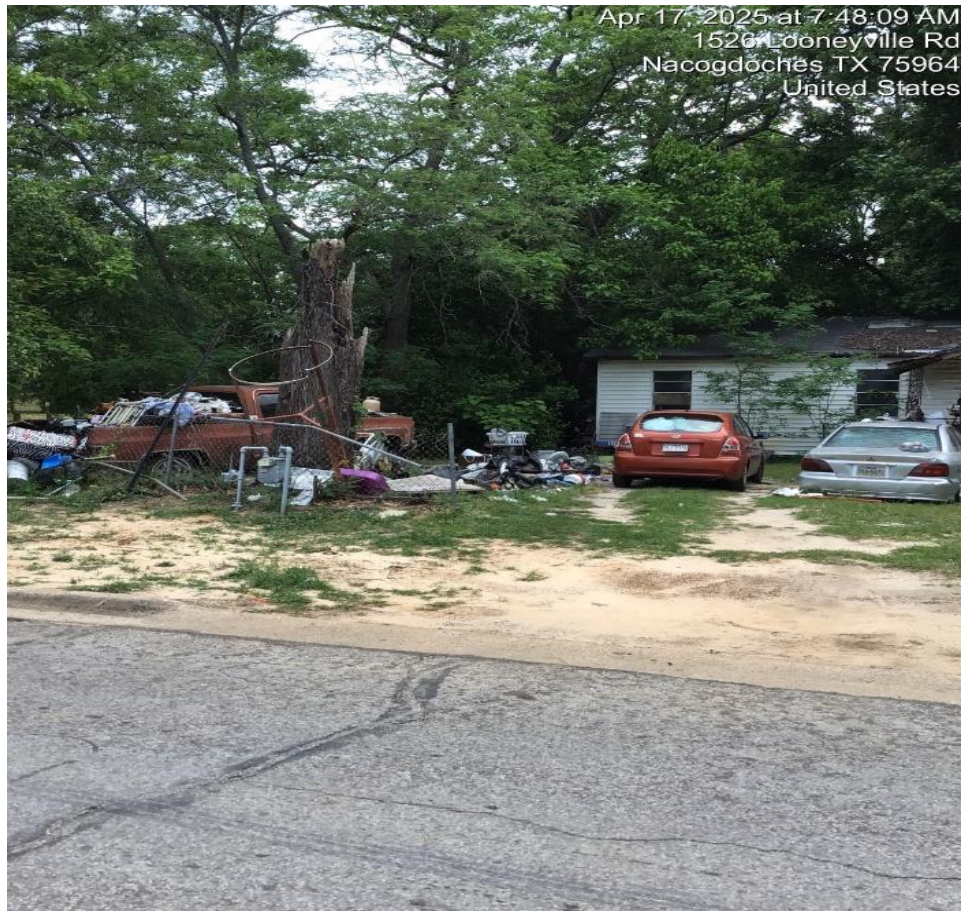
View of structure showing rubbish. Photo taken April 17, 2025.
