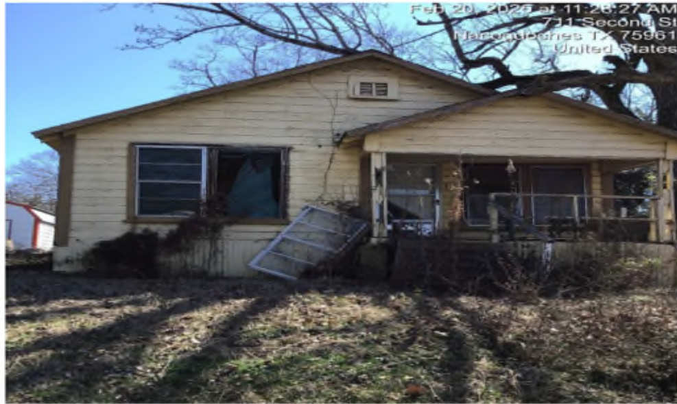
View of structure frontage. Photo taken February 20, 2025.
