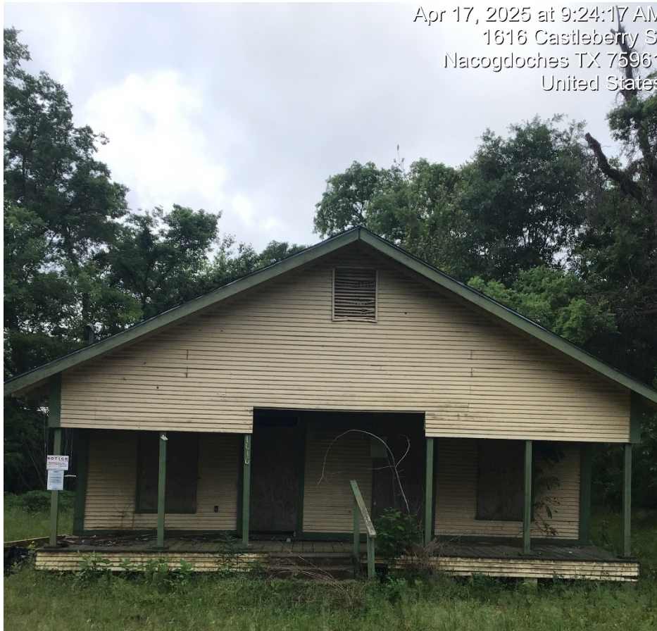
View of structure showing notice posted. Photo taken April 17, 2025.
