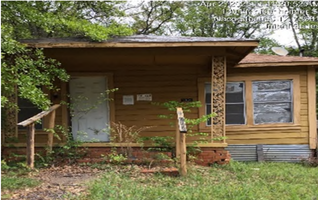
View of structure showing posted notice. Photo taken April 2, 2025.
