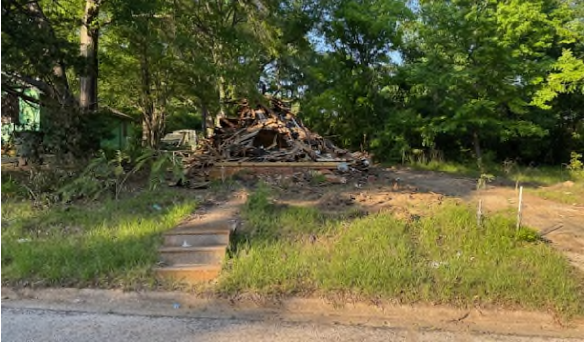
View of structure showing debris from supposed demolition. Photo taken April 16, 2025.
