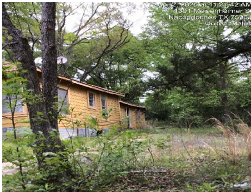
View of side of structure. Photo taken April 2, 2025.
